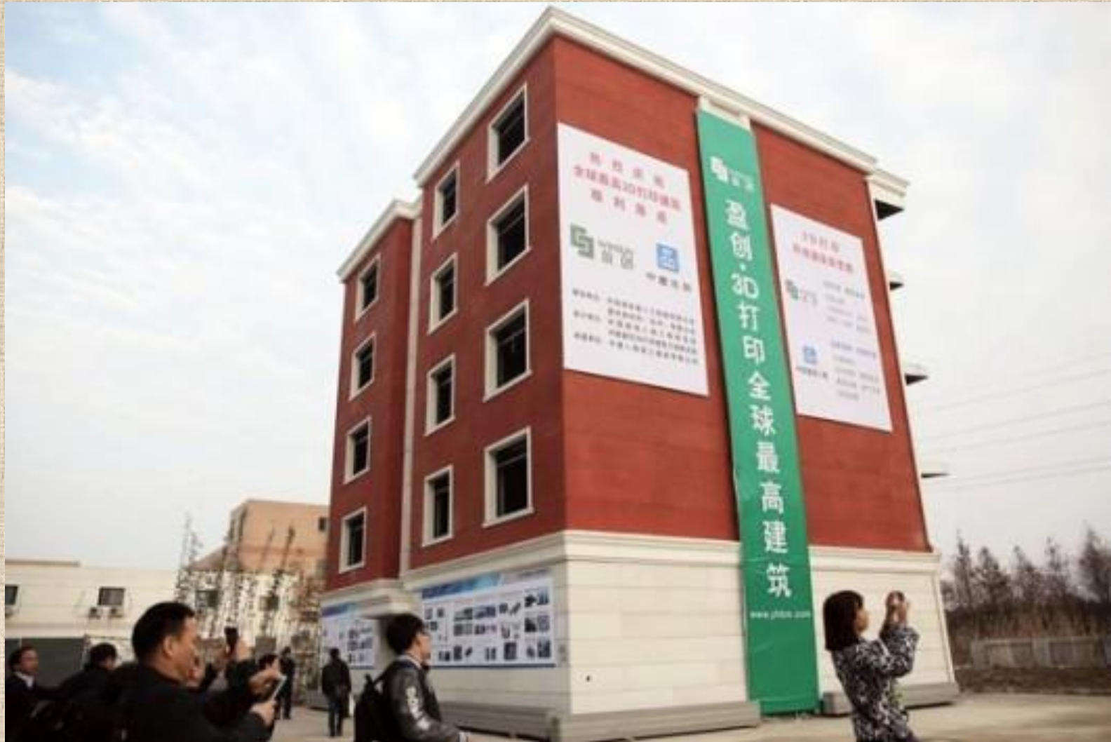
3D Printed Building (China)
